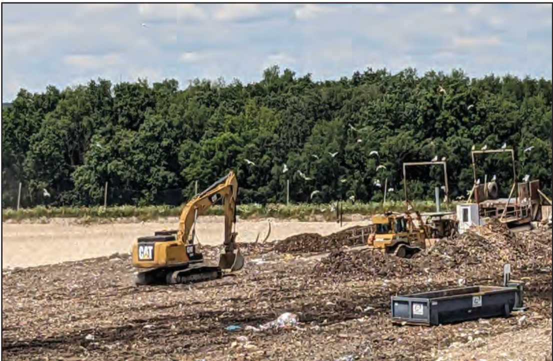
Working face covering for the day
