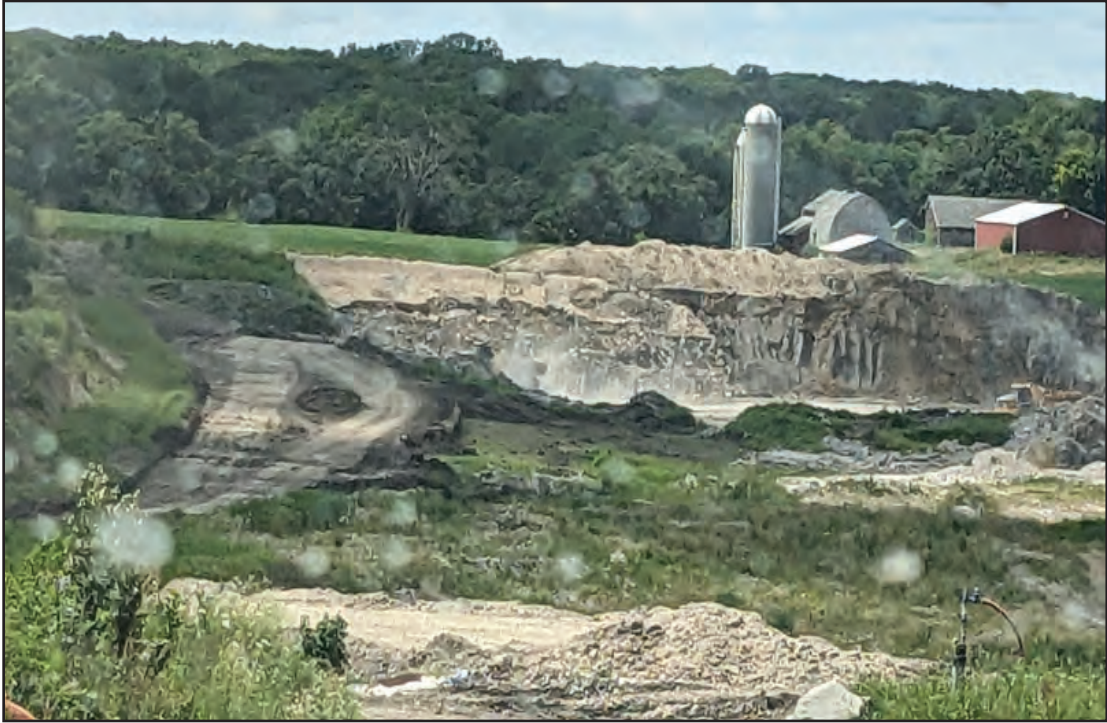
Borrow area providing clay for cap over plastic cap placement
