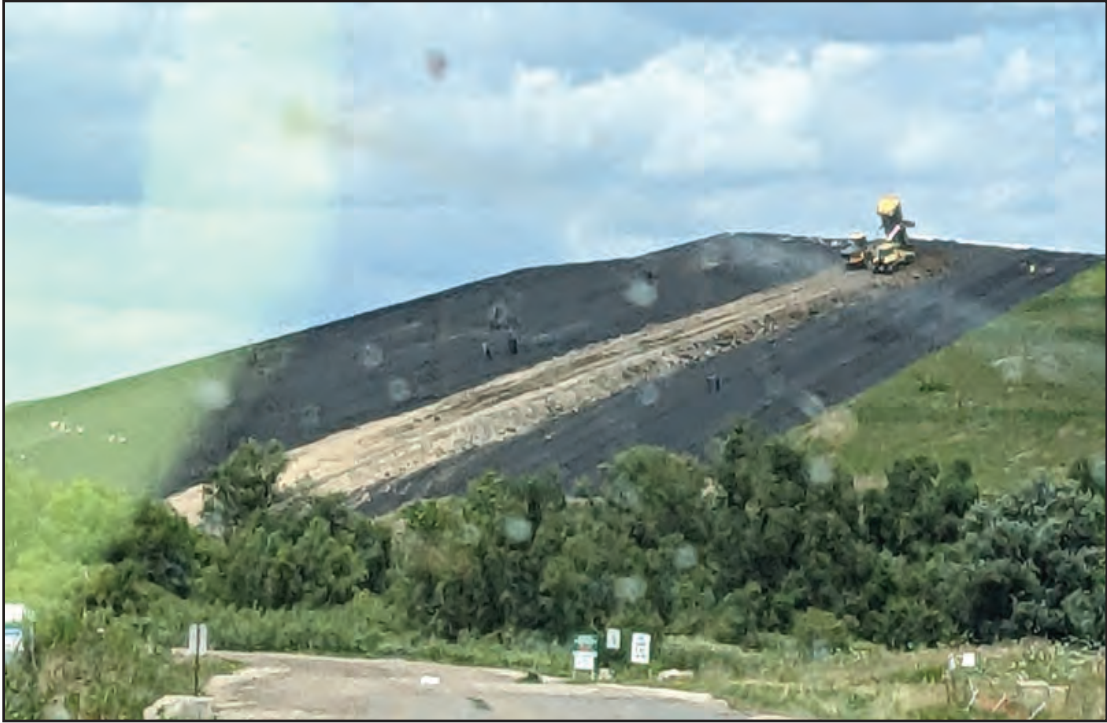
Soil pushed ahead of equipment to protect cap
