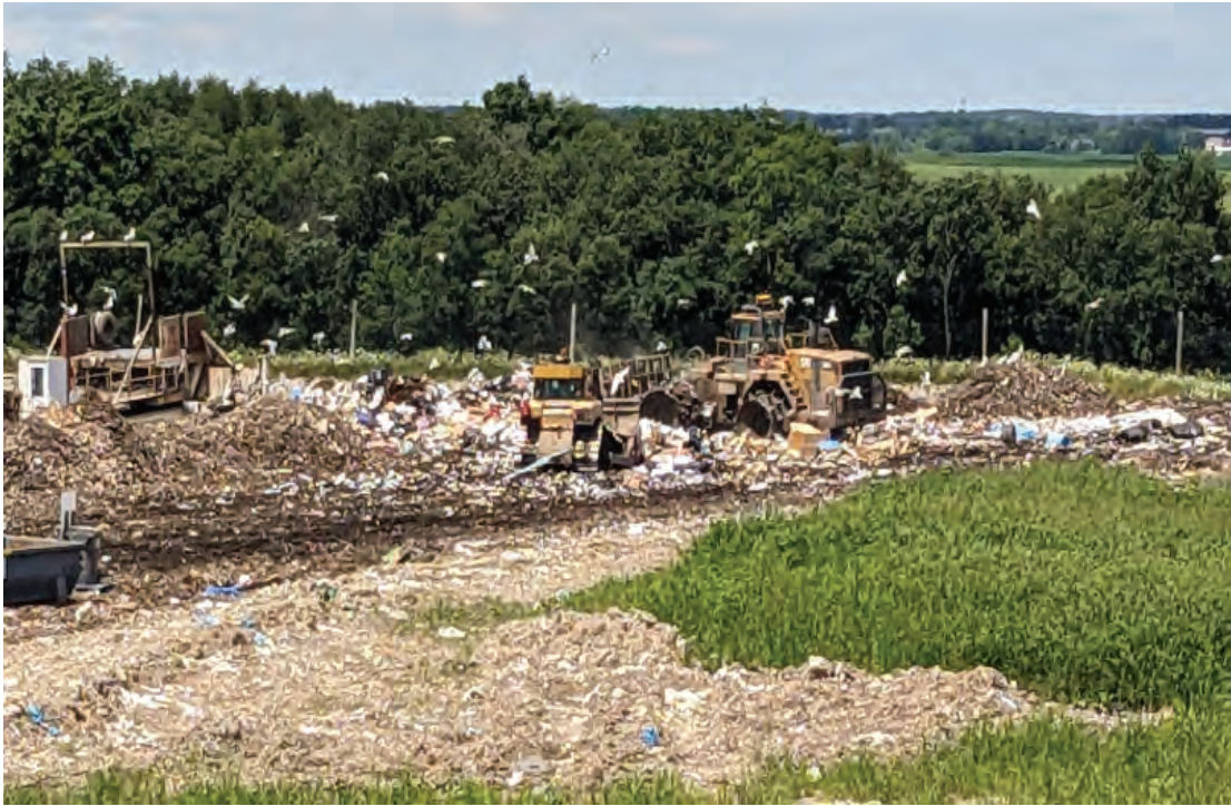
Working face covering for the day
