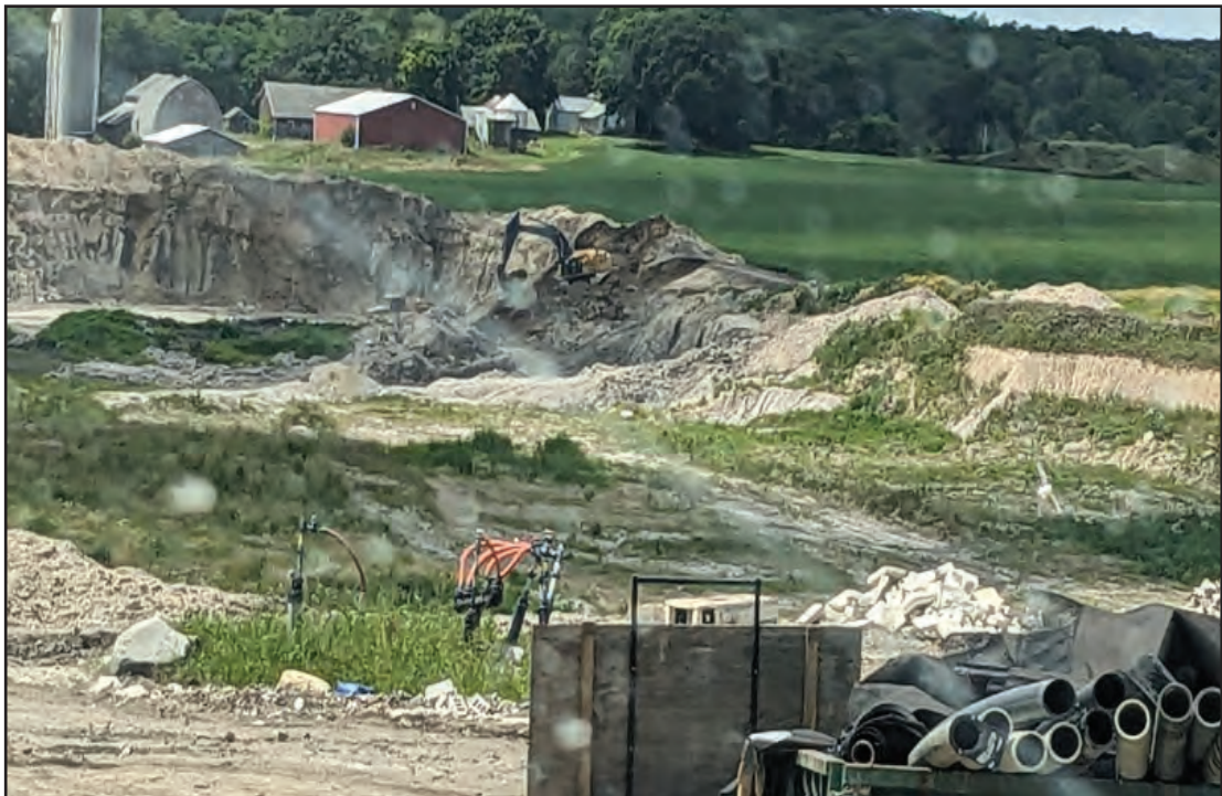
Borrow area providing clay for cap over plastic cap placement
