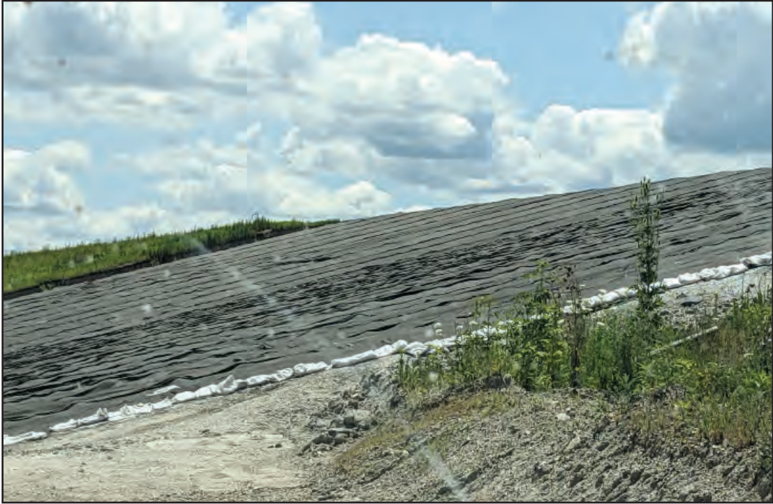
Plastic cap and geocomposite awaiting more clay on East slope on mass
