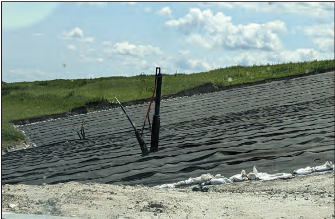
Plastic cap and geocomposite awaiting more clay on East slope on mass
